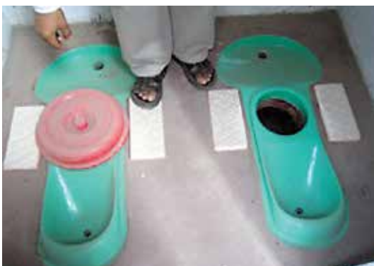
Ecosan toilets in Musiri, India. The left side collects feces, and the right side collects urine.
